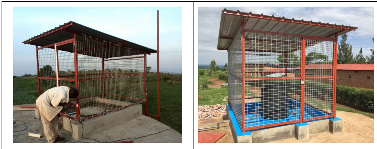
Figure 11: Construction of roof structure
