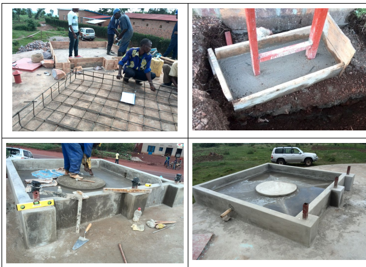
Figure 10: Construction base concrete
