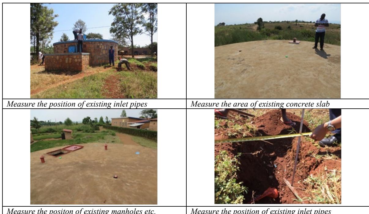
Figure 1: Measurement of the dimension of the existing reservoir
