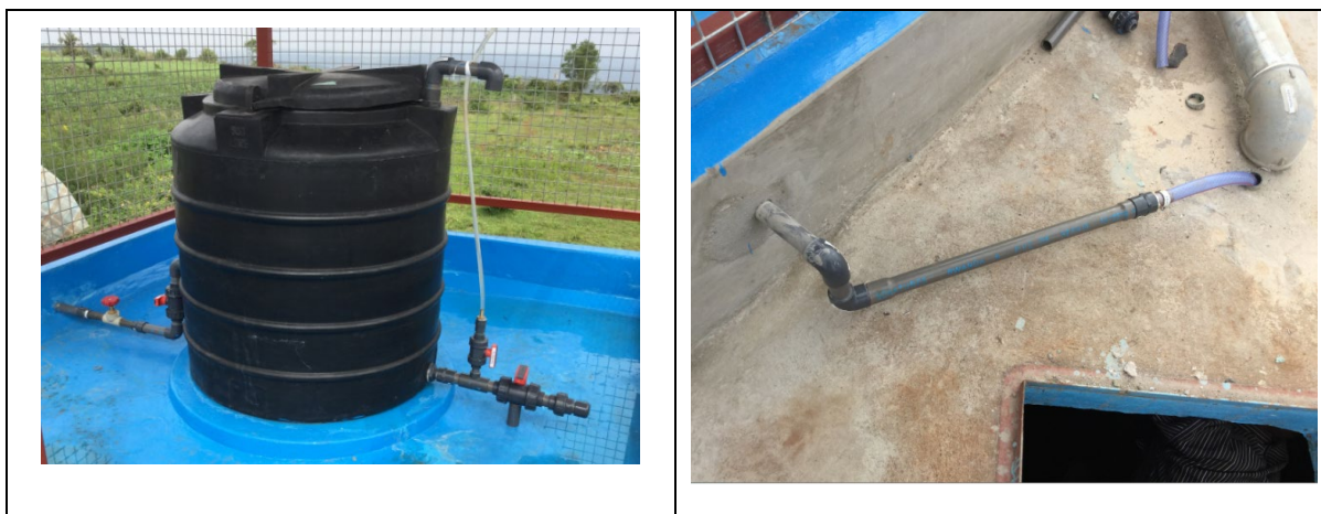
Figure 12: Installation of storage tank
